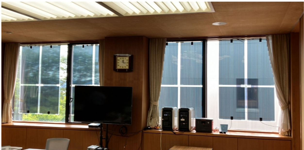
ST-OPV installed in the Mayor's Office at Nakafurano Town Hall
